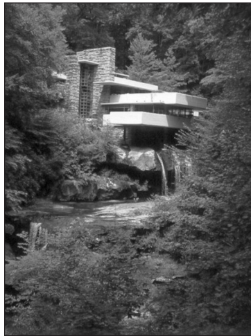
Figura 3 FALLINGWATER, FRANK LLOYD WRIGHT, 1935
